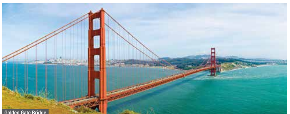
Golden Gate Bridge
